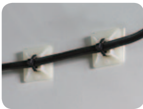
Inside the control panel
