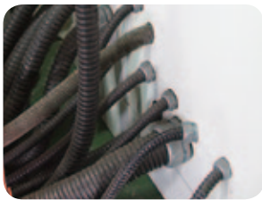
Outside the control panel
